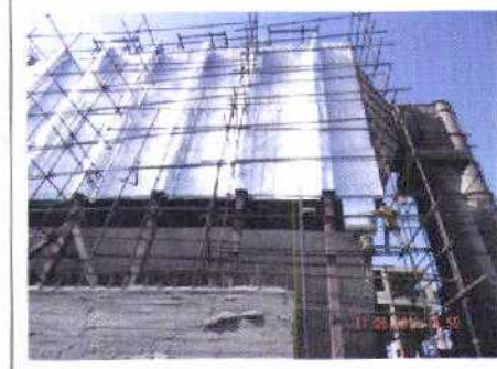
BMR Equipment in its Installation Phase
