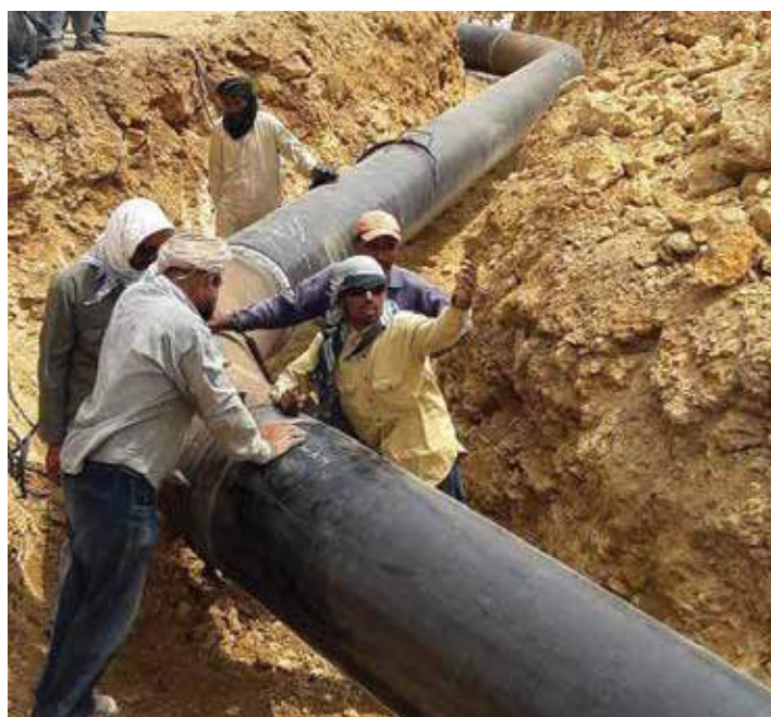
Winding paths: A pipeline construction activity in progress
