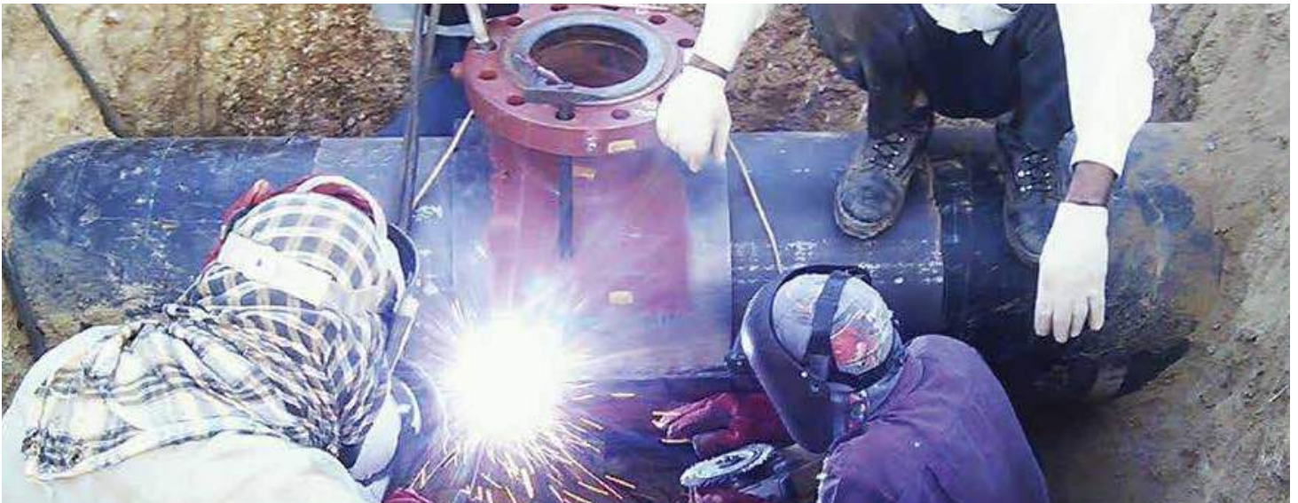
Countering UFG: SSGC team undertaking a pipeline rehabilitation activity in Karachi
