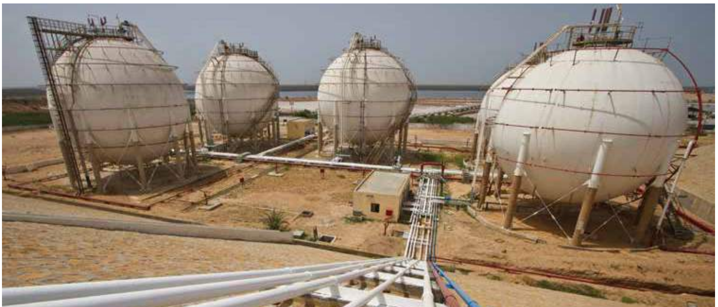
Positive Change: A view of SSGC-LPG Terminal in Port Qasim, Karachi
