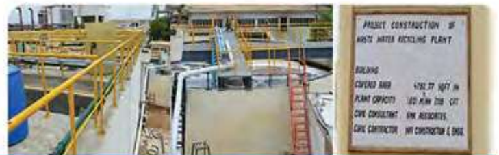
Waste water treatment and recycling plant
