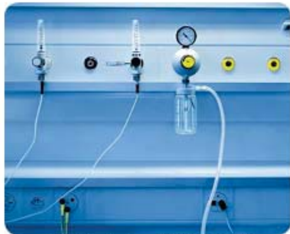
Complete bedhead panels installed at hospital
