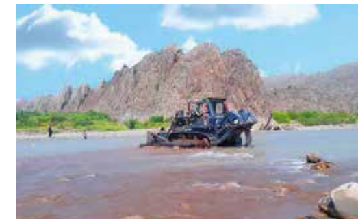
Dozer Operation in challenging terrains
