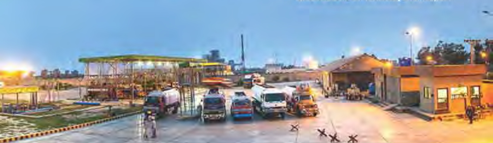
Machike Bulk Oil Terminal, Sheikhupura
