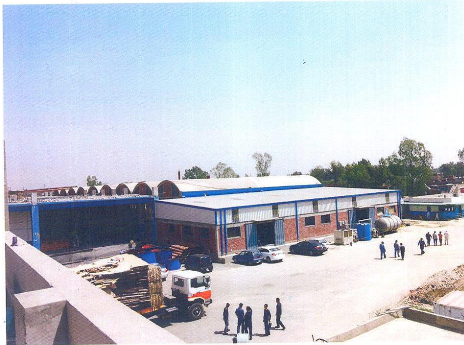
Civil Work – Corrugation Extension [ANNEXURE-B]
