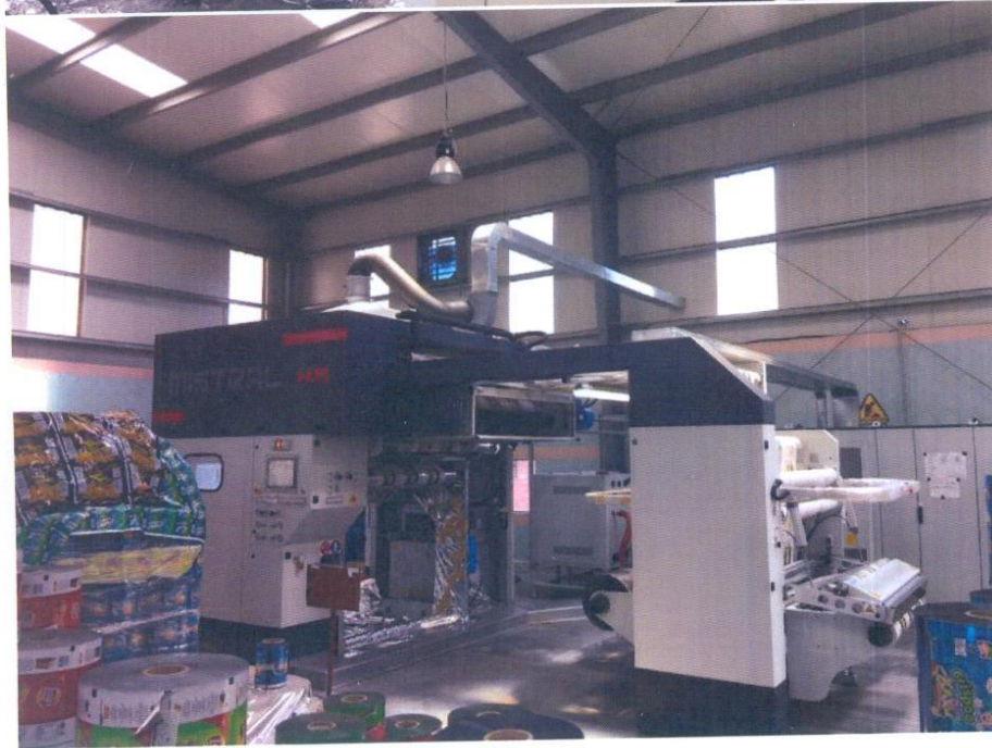
Converting Hall – Flexible [ANNEXURE-G]
