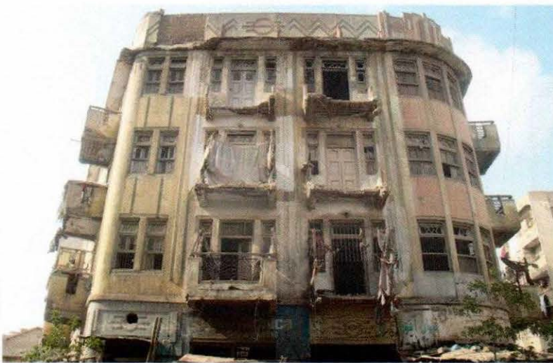
KARACHI: A decaying building at Ath Chowk needs attention of authorities.—Online
