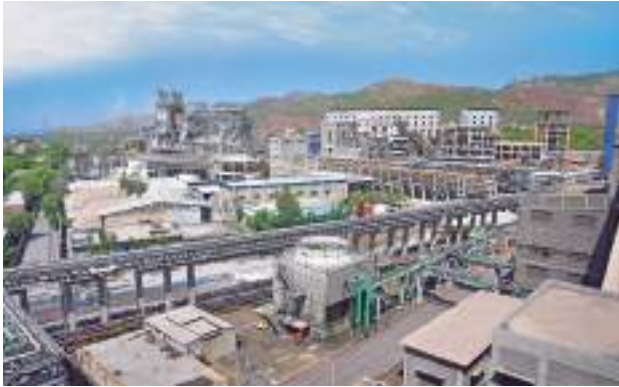
The Phase 2 of 150,000 tonnes per annum Light Ash capacity expansion at the Soda Ash Plant, being expansion of 75,000 tonnes per annum, is now underway
