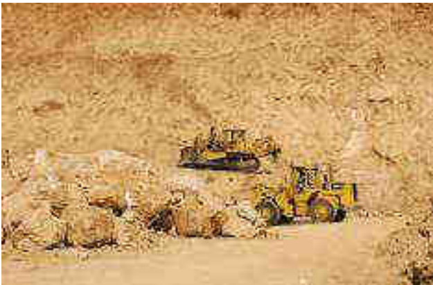
LIME STONE QUARRY
